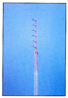
The top section of the 660-foot tower after the FM antenna was mounted.
